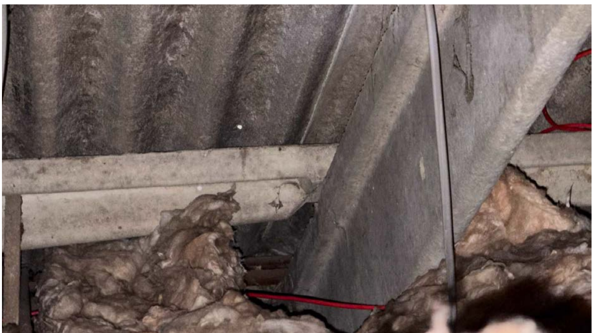
Daylight through roof panels.
